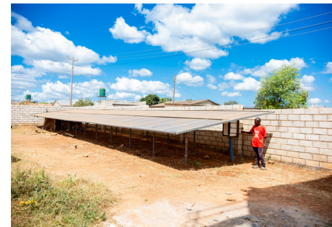
A technician in Gondwe, Lusaka, Zambia, shows solar panels that power a new water distribution system, including a borehole and water tower. The system now provides reliable, clean water to residents of this low-income community, who previously had to rely on the goodwill of others. @WSUP/Charles Mulomba
