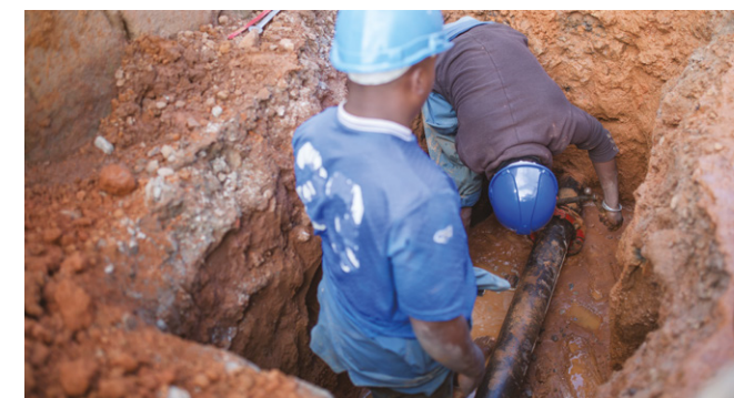
JIRAMA, Madagascar's state electricity and water utility, has a Non-Revenue Water (NRW) reduction team in Antananarivo that works with WSUP to cut water losses, a critical step in improving the utility's efficiency and financial sustainability. ©WSUP/Tsilavo Rapiera
