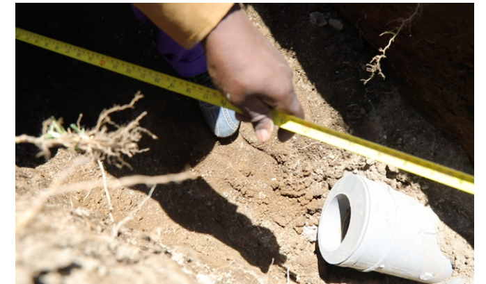
A technician installs pipes for a simplified sewer system, providing an affordable, effective solution to bring safe, resilient sanitation to low-income urban communities and informal settlements. @WSUP/ Awaken Pictures
